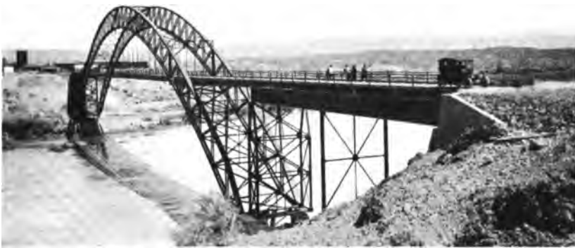
Perspective view of same bridge from the California side of Colorado River.
